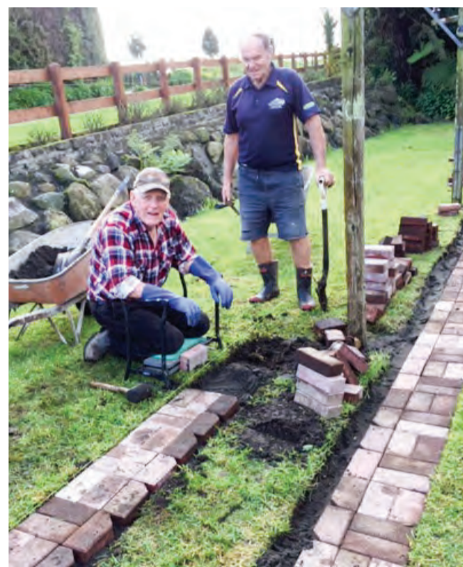
Gib Baxter and Andy Davy laying bricks.
